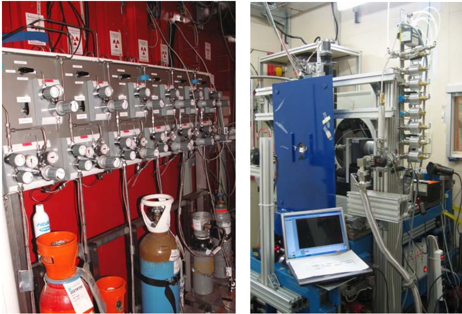
Figure 10. The array of gas bottles outside the experiment hutches, and the gas mixing system designed for high gas pressures installed on the MAR345 image plate setup
